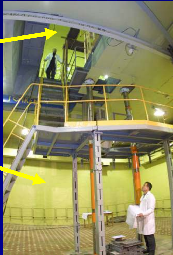
Installation of the supporting elements for a new linac
