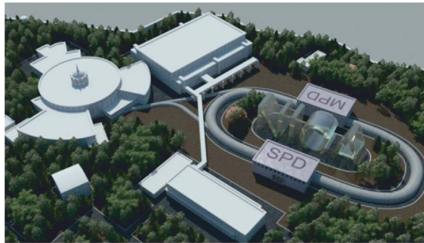
Fig. 5. The location of MPD and SPD detectors at the NICA collider complex
